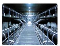
Fig. 1: View of pipe installation walkway with DN 1000, DN 1200 and DN 1400 pipelines
